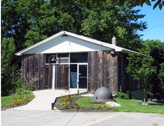
The former “Agriculture Building” alone will provide close to 1,800 square feet of additional space .
